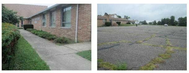
Parking spots can be replaced with porous asphalt to capture and infiltrate stormwater runoff from the parking lot. Two rain gardens adjacent to the building can capture, treat, and infiltrate roof runoff. A preliminary soil assessment suggests that more soil testing would be required before determining the soil's suitability for green infrastructure.
