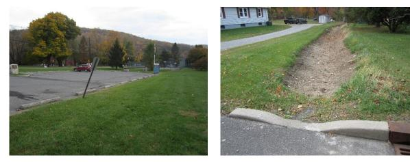
Rain gardens can be installed to capture, treat, and infiltrate runoff from the parking lot and roadway. A bioswale can be built in the ditch to the south of the basketball court to intercept runoff before it reaches the catch basins. A preliminary soil assessment suggests that more soil testing would be required before determining the soil's suitability for green infrastructure.
