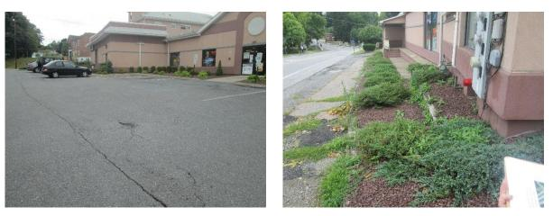
Parking spots to the northwest lot of the building can be replaced with porous asphalt to capture and infiltrate stormwater. Stormwater planters along the southeast side can capture and treat roadway runoff. A preliminary soil assessment suggests that more soil testing would be required before determining the soil's suitability for green infrastructure.
