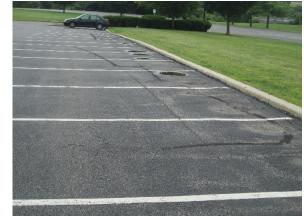
Parking spots to the west of the building can be replaced with porous asphalt to capture and infiltrate stormwater. A rain garden can be installed in front of the building to capture, treat, and infiltrate rooftop runoff. A preliminary soil assessment suggests that the soils have suitable drainage characteristics for green infrastructure.
